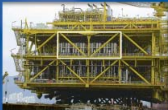
16" membranes at CTOC's 700 MMscfd Cakerawala platform in the Gulf of Thailand
